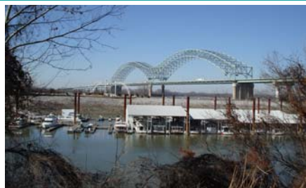
HEPACO begins work on the Hernando DeSoto Bridge over the Mississippi River.
