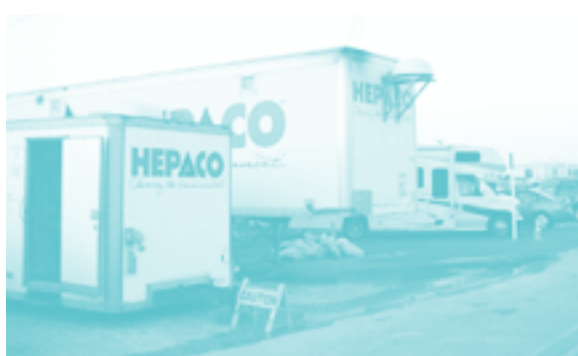
HEPACO's command post and decontamination trailer in Gulfport, MS, serve as home base for post-Katrina cleanup efforts, including removal of debris from runways and decontamination of a tower for the Federal Aviation Administration (FAA).
